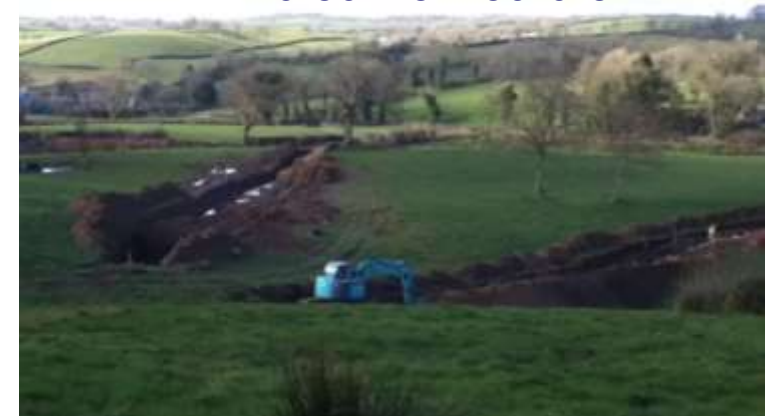
TRENCHING AT CLAY LAKE
